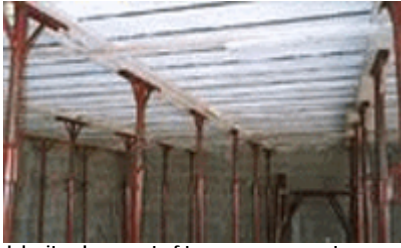
Job site placement of temporary supports
